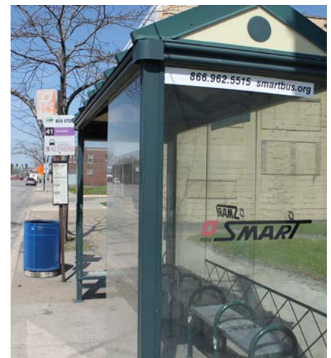
Bus shelter for bus line 41
