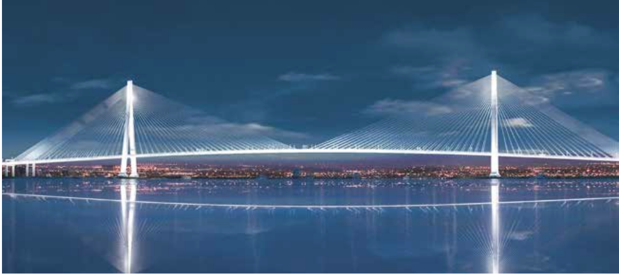
Visualization of the future Gordie Howe Bridge in Detroit about 2 miles from River Rouge.
