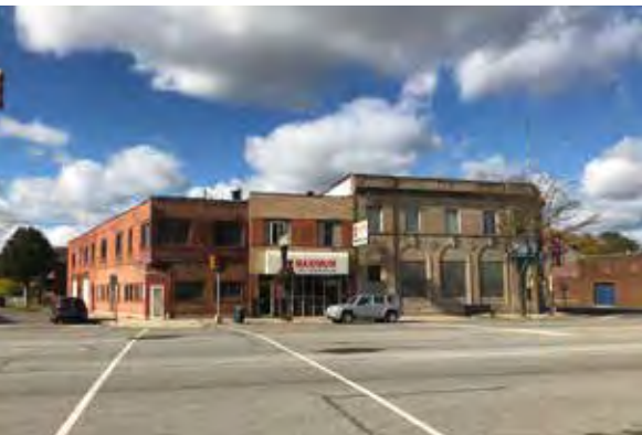
Vacant building on Jefferson Avenue provide opportunity for reinvestment.
