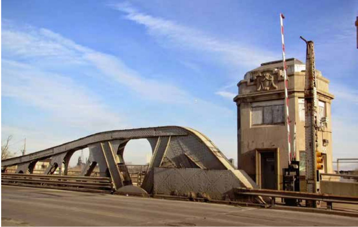
W. Jefferson Avenue Drawbridge over Rouge River.
