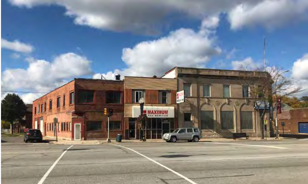
Commercial storefronts along Jefferson Avenue in River Rouge.
