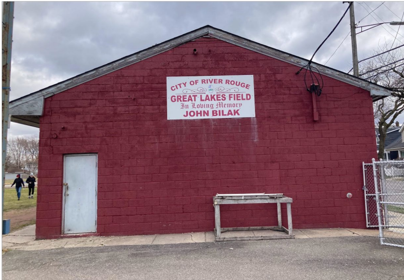
Equipment building at Great Lakes Field.
