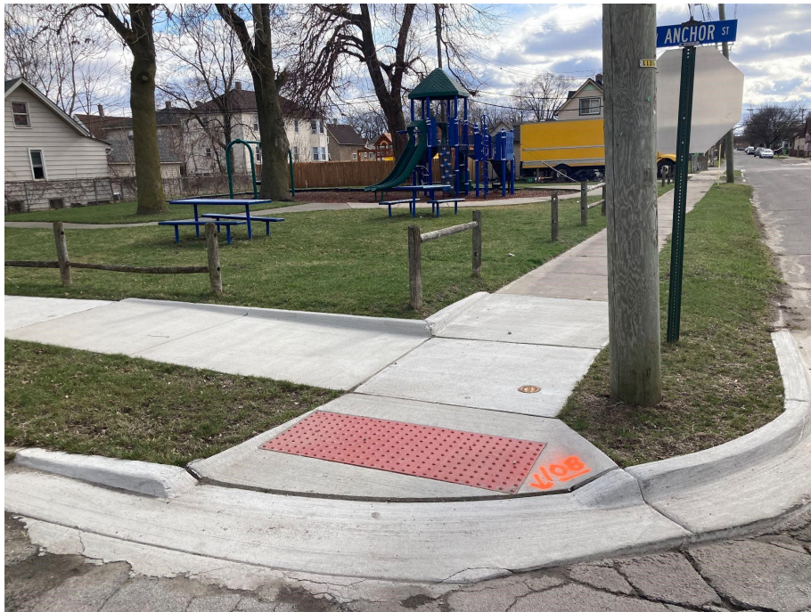
Division & Anchor Tot Lot from street view.
