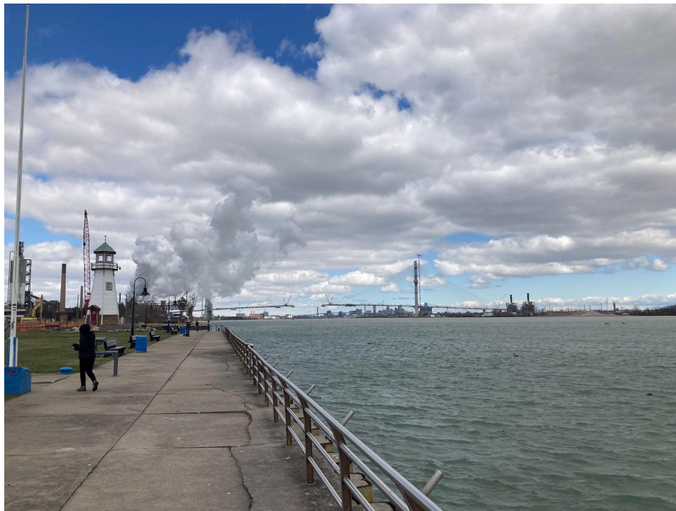
Waterfront view from Belanger Park, including the construction of the Gordie Howe Bridge.
